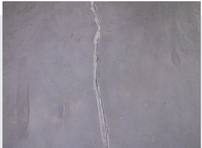
Crack prepared and ready for treatment
