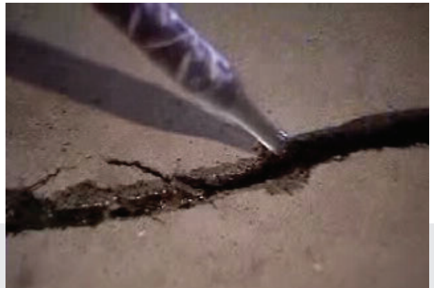
Saturate the Crack with CLF Rapid Repair Fixcrete.
