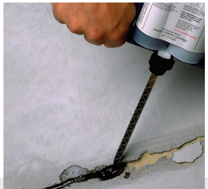
Rapid Repair Fixcrete deep penetration.
