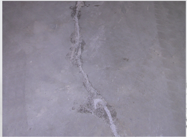
Crack after repair
