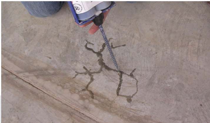
Repair of Surface Delamination.
